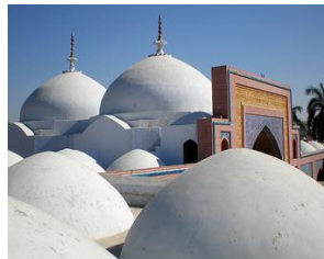
Fig. 2.6 An outside view of the domes of Shahjehani Mosque Thatta
